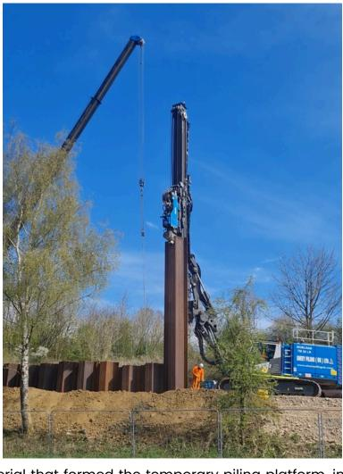
We are now in the process of removing the material that formed the temporary piling platform, in preparation for the next stage of road reconstruction. This will include trimming the area to subbase level in readiness for the final surfacing layer. We will also be installing rear wall filter drainage along the sheet pile wall. The next steps will involve applying road markings, installing fencing along the sheet pile wall and the installation of ground monitoring equipment.
